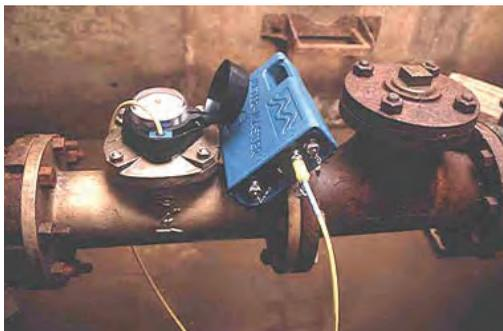
Meter-Master flow recorder installed on a magnetic drive water meter.
